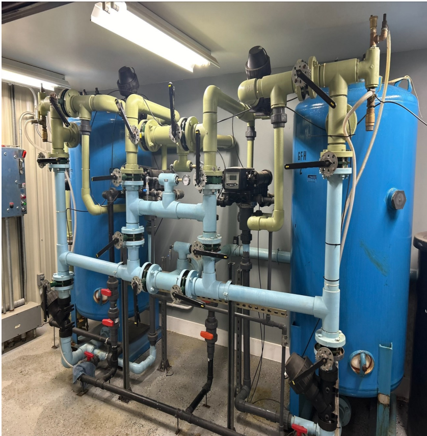
Grindstone Arsenic Removal Media Vessels
